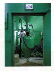
A pneumatic pressure vessel conveyor automatically supplies the sanding stations with brake sand from the storage silo via the pneumatic conveying pipe. The gentle plugflow conveyance preserves the grain structure of the sand and prevents the generation of dust.
